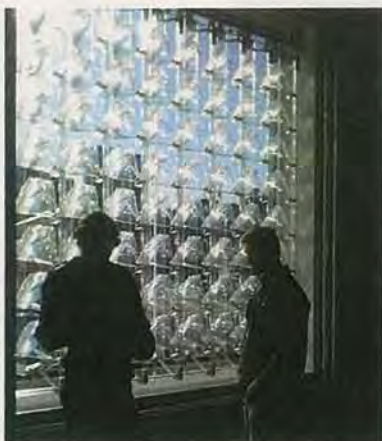
The solar facade: concentrators hung on wires that move up and down and twist side to side.
